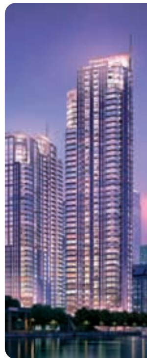
Pan Peninsula, the UK's largest residential building, will use a CHP installation from Ener-G Combined Power to produce 135kW of electricity and 215kW of heat
